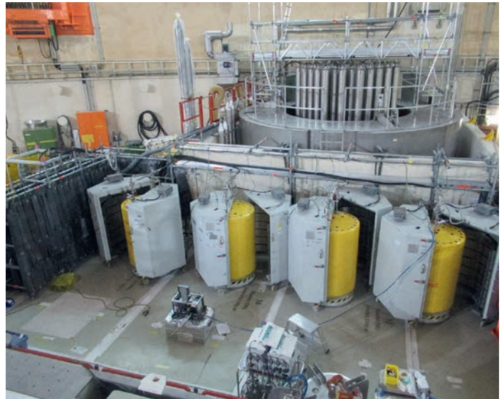
Drying of the loaded MOSAIK® casks with the GNS facility KETRA.
