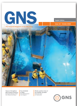
ZerKon project: dismantling of the RPV internals at Grafenrheinfeld NPP.
