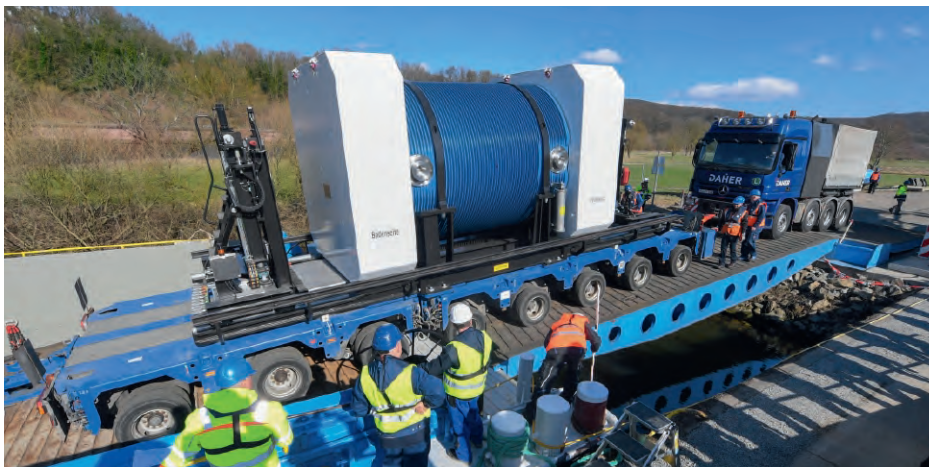
First functional test in February 2017: In Obrigheim, an unloaded CASTOR® cask is driven on a universal transport frame on to the transport vessel. (Picture: EnBW Kernkraft GmbH)
