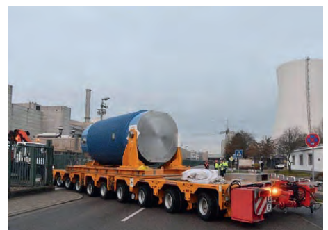
The 17th CASTOR® V/52 with the last FAs of KKP 1 on their way to the KKP on-site storage facility.
