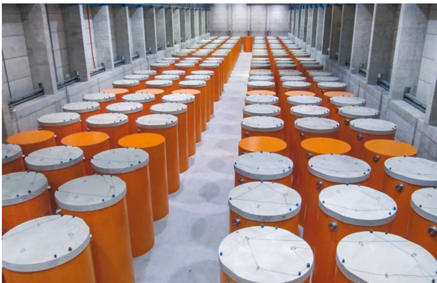
View into the full Interim Spent Fuel Storage Facility (ISFSF) in Ignalina: The CONSTOR® casks with additional protection plate are already loaded.
