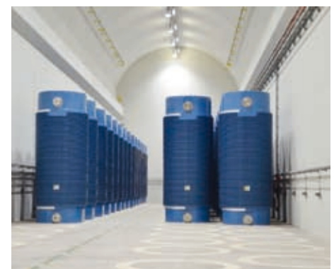
Tunnel storage facility in Neckarwestheim. Photo: EnBW
