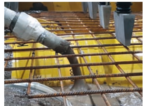
Concreting with hold-down device.
