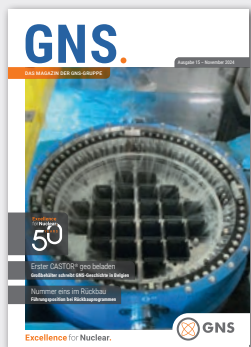
Loading of the first CASTOR® geo at the Belgian nuclear power plant Doel.
