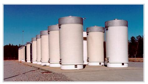
Fig. 5. CASTOR<sup>®</sup> V/21 casks at Surry nuclear power station, Virginia/USA.
