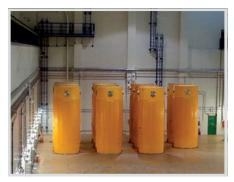
Fig. 7. CASTOR<sup>®</sup> 1000/19 in the interim storage facility at Temelin/Czech Republic.
